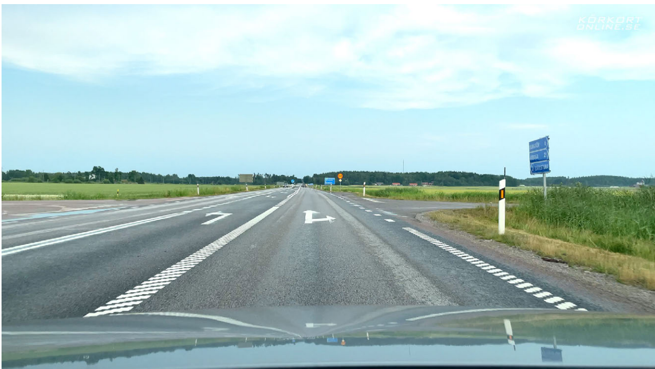
The verge post on the right has a yellow reflector to mark the junction.
