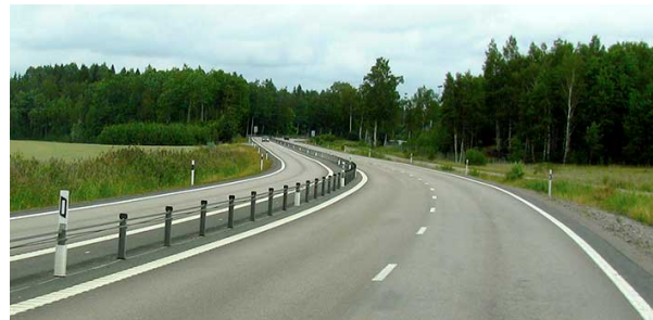
A 2+1 road with cable barriers.
