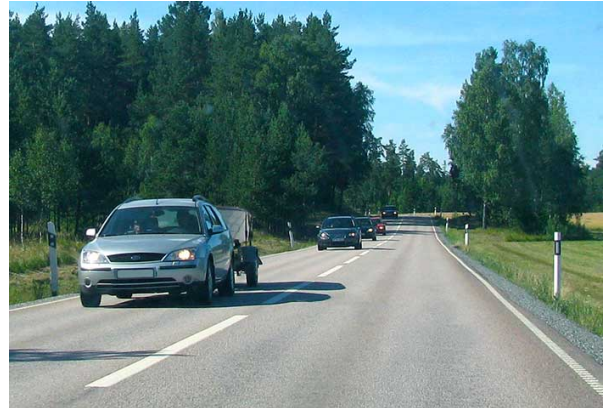
The distance is insufficient. Note the verge posts.
